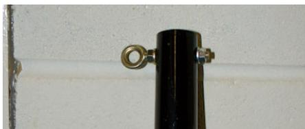
**Figure 14 - Boom With Eyebolt Installed**
