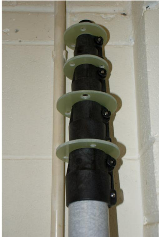
**Figure 15 - Mast With Guy Rings Installed**
